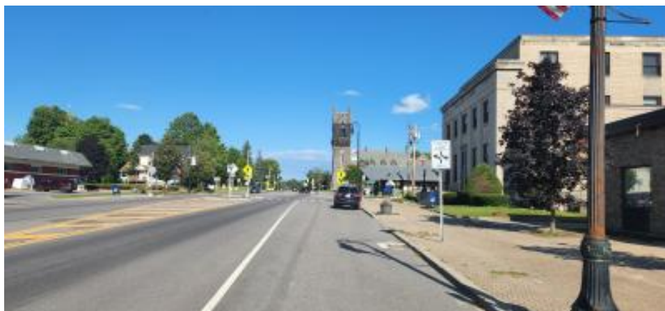
Opportunity for Road diet: This section of Route 11 is very wide with a center pedestrian island and very wide shoulders. Buildings set back off the road and lack of street trees and other amenities in this location illustrates the opportunity for an improved streetscape and a 'road diet' to create a safer and more pedestrian-friendly atmosphere.
